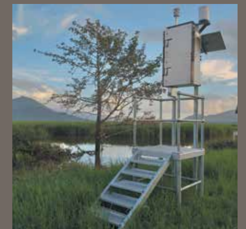
In-situ monitoring infrastructure
