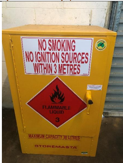
Figure 2 Flammable chemicals cabinet
